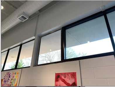
Existing painted clear anodized storefront adjacent to new dark bronze anodized storefront
